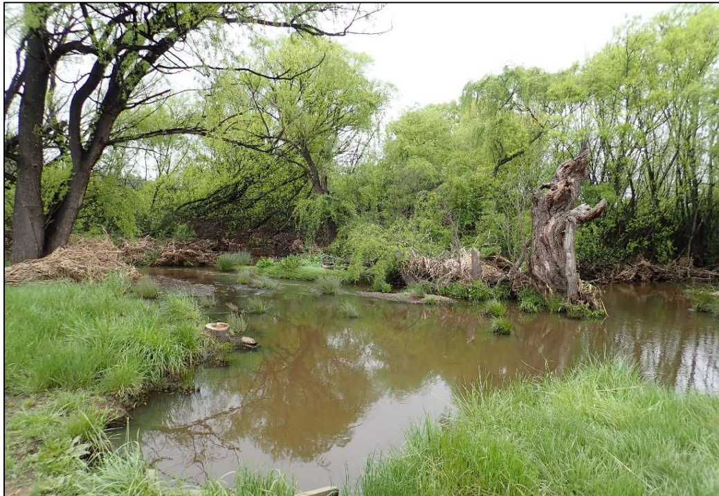
Willows and privet have been removed to clear the area for planting. Stumps are left to help stabilise the creek bed. Some willows will be left as shade trees. Selective weed spraying on the banks will help prepare for native planting.
