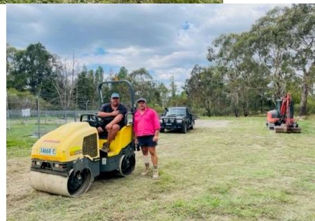
Preparing the new site. Images: Kerry Steller
